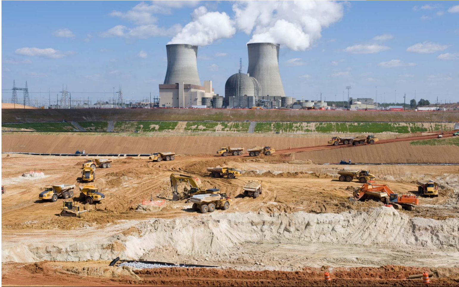
Plant Vogtle Unit 4 foundation excavation showing Unit 1 and 2 in background with water vapor rising from cooling towers. March 4th, 2010.
